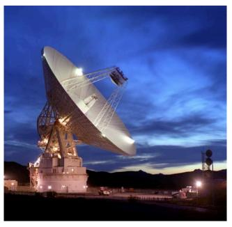
Two or more widely spaced radio telescopes are better than one — the combined output is like that of a telescope as large as the distance between the two.
