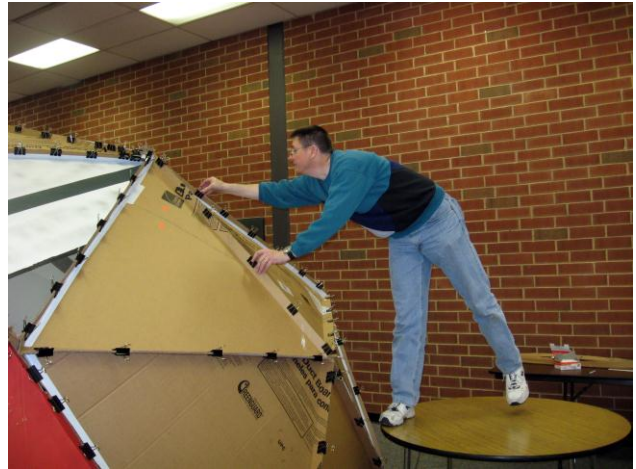
Mark Brown attaches binder clips to secure the structure of the Fendrich Planetarium. Photo by Jean Fendrich.
