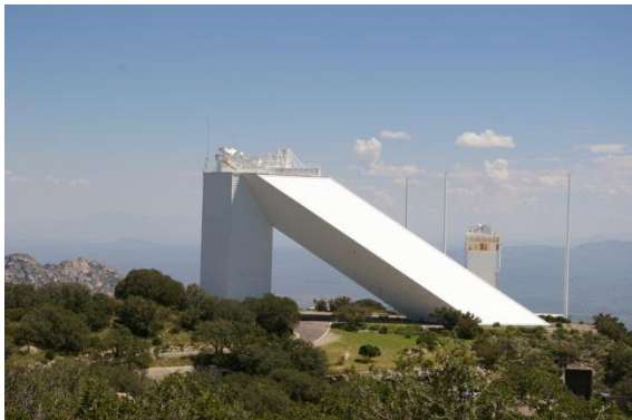
The McMath-Pierce Solar Telescope. A mirror can be seen on top that follows the Sun across the sky and reflects its light down the telescope building. Photo by Bill Breedon.
