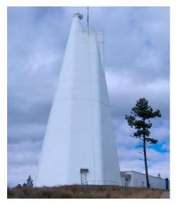
The Richard B. Dunn Solar Telescope extends from 136 ft. above ground to 228 ft. below through a series of mirrors in a vacuum throughout.
